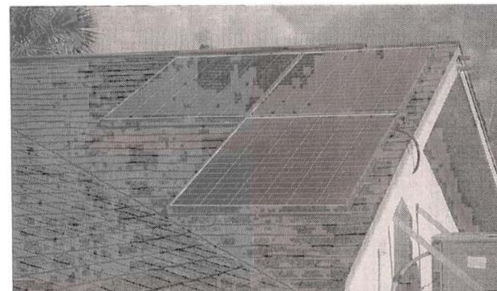
Three photovoltaic solar panels generate enough free electricity to run homeowners' swimming pool filters from sunup to sundown, saving hundreds of dollars per year.
